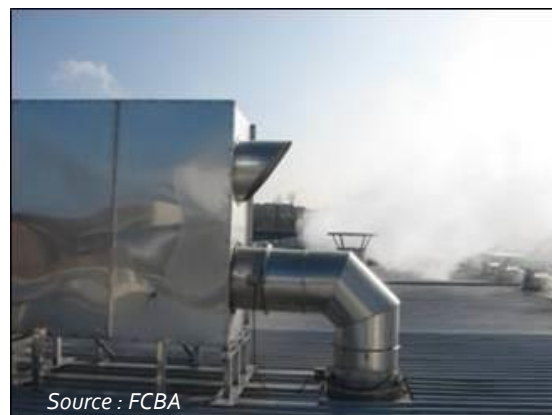
Heat recovery unit of a drier
